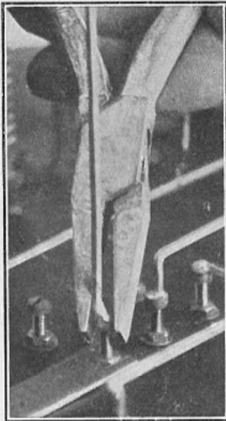
Fig. 11. Tightening the Terminal Nuts (note flat spanner bottom left).
